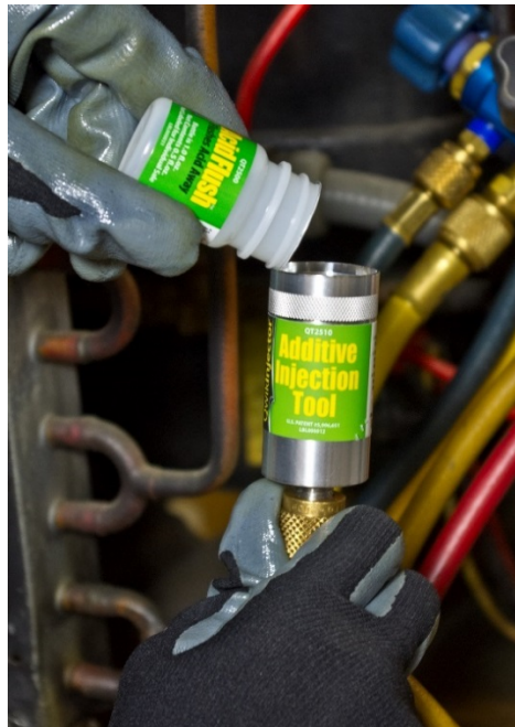
Figure C-12. QwikShot® added to a system with a QwikInjector®
