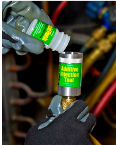
Figure 17. Adding QwikShot® to QwikInjector® for use
